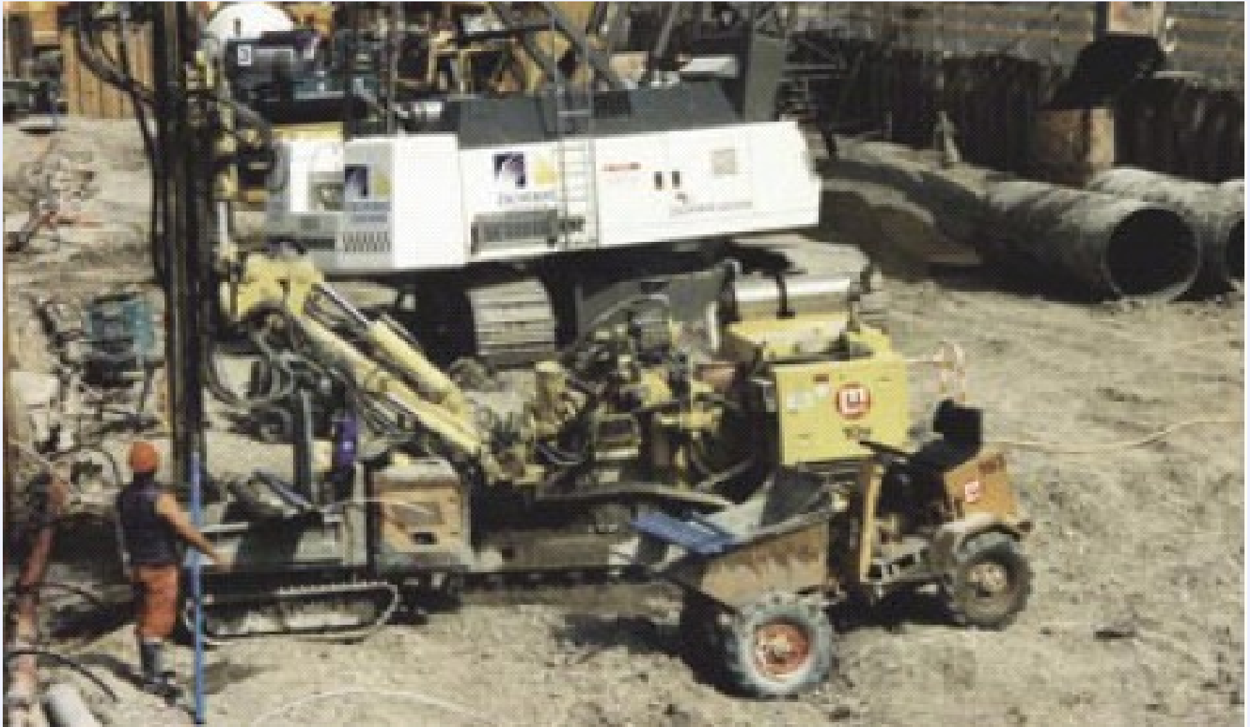
Construction work –mainly in urban areas
